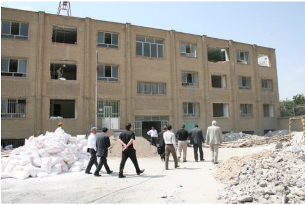
Seismic retrofitting of a school building, Tehran.
